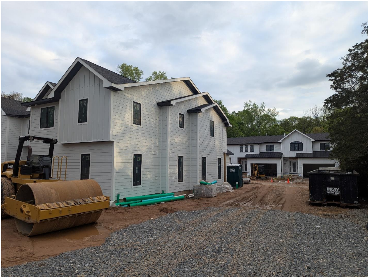
Photo 1 - Progress of 95 County Road Inclusionary Development as of May 7, 2025
