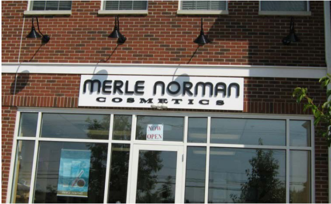
(3) Individual cut letters with gooseneck lighting. Example below.
